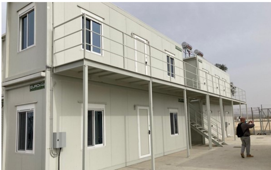
Figure 22. Block of 4 containers on 2 floors, capacity of 16 (Safe Zone, Pournara First Reception Centre, Cyprus)
